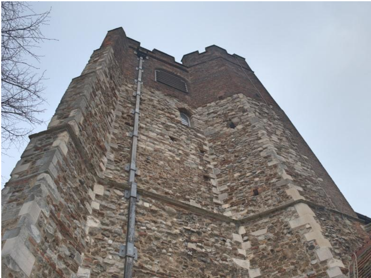
Figure 7: St Mary at the Wall. Note the different brick at the top which shows the eighteenth-century repairs (Picture: author's own).
